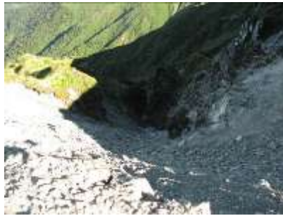
Steep eroded edges
