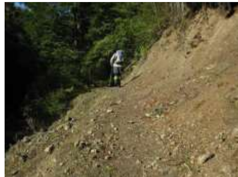
Minor landslip zone
